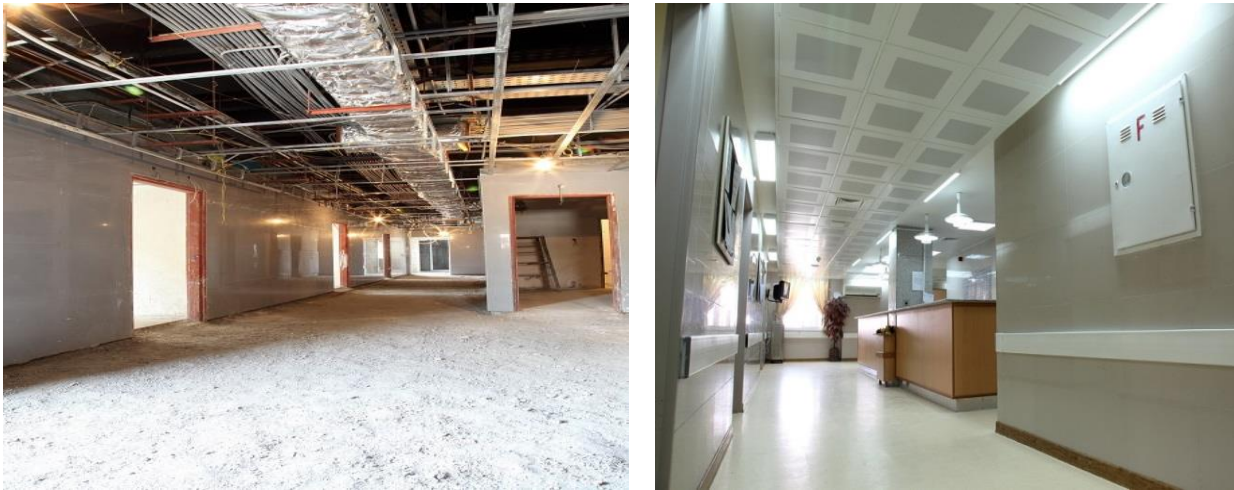
Figure 12. A view of the project before and after installing false ceiling
