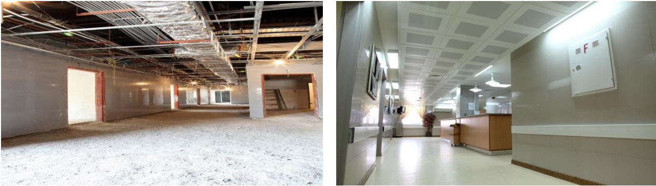
Figure 23. The project before and after installing the false ceilings
